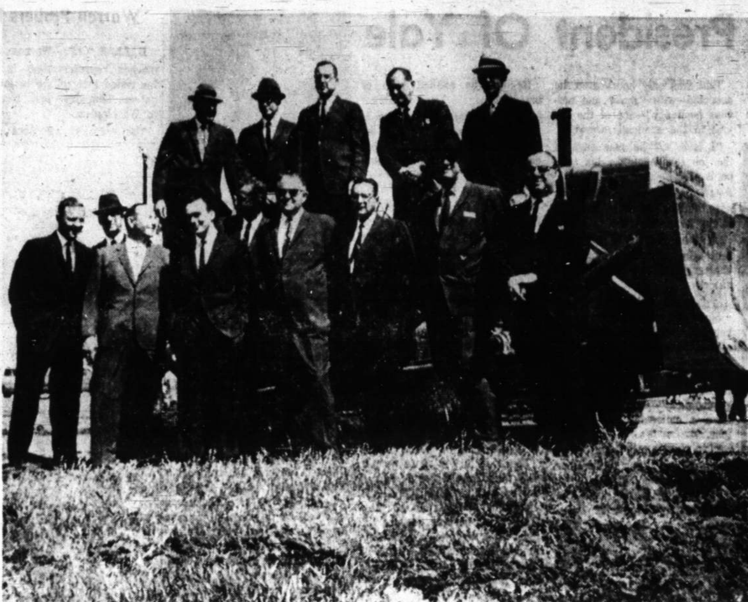
IMPOSING LOAD—Directors of the new Southwest National Bank climbed aboard and stood at side of the bulldozer which pushed down the last tree Friday morning on the bank site on FM 369 a short distance west of Fairway. Above are, left to right, top row, Bill Thompson, Jimmie Whit-
