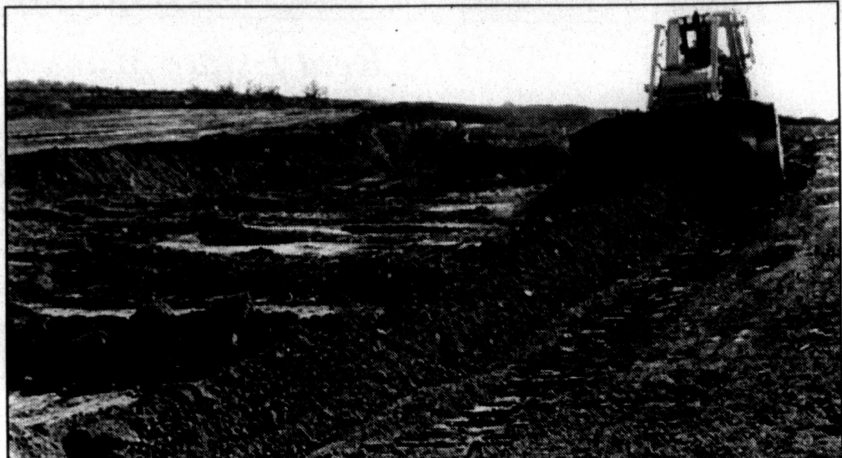
FOUR-T CONSTRUCTION CO. of Christoval is currently working on the water treatment, above, and water storage lagoons at Loraine's new wastewater treatment plant north of I-20. Ricky Bailey, water superintendent and public works director, said the treatment lagoon measures 300 feet by 150 feet while the storage lagoon measures 500 feet by 300 feet. The lagoons cover 5 acres while the main operation will be located on 70 acres. Four-T submitted the low bid of $437,587.98.
