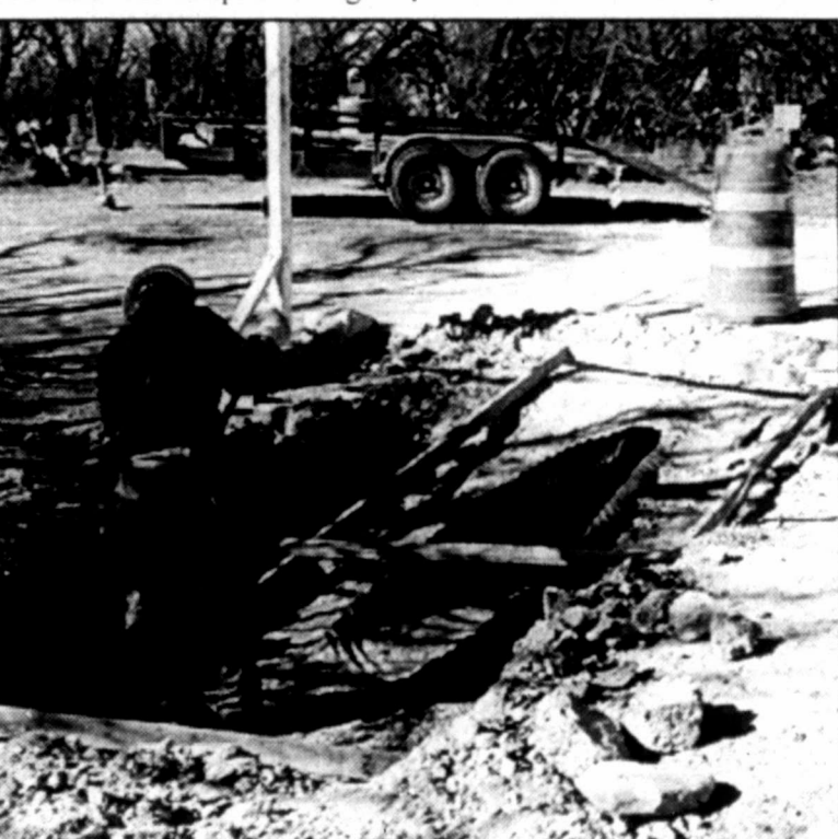
REECE ALBERT CONSTRUCTION of San Angelo is nearing completion on the third section on the north part of the Farm-to-Market Road 644 project north of Loraine. Roy Dill, area engineer at TxDOT's Big Spring office, said culverts are being constructed in the area while he expects the riding surface to be laid within two weeks. The project then moves to FM 644 south of I-20, involving 2 1/2 miles of road.
