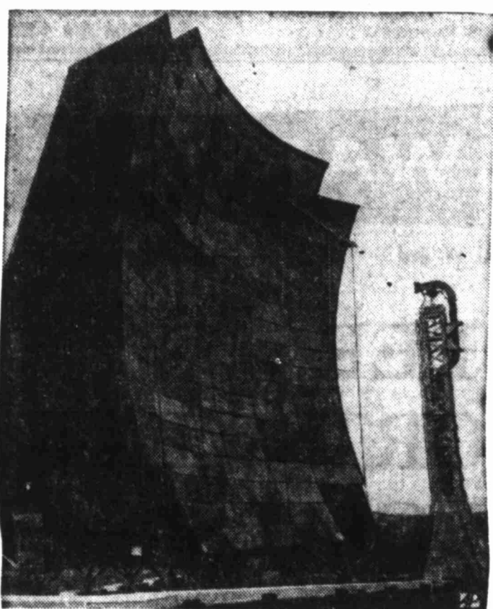
COLD PACK — Workmen caulk seams of face of 60-foot parabolic antenna, one of the "iron ears" of communications system that stretches 3,100 miles across Alaska.
