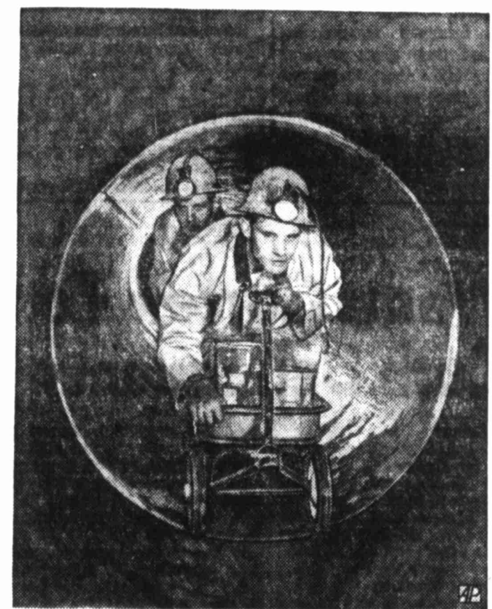
PIPE ROLL — Workmen use a toy wagon to transport their tools and materials through 48-inch diameter pipe tunnel being completed for Pittsburgh's sewage system.
