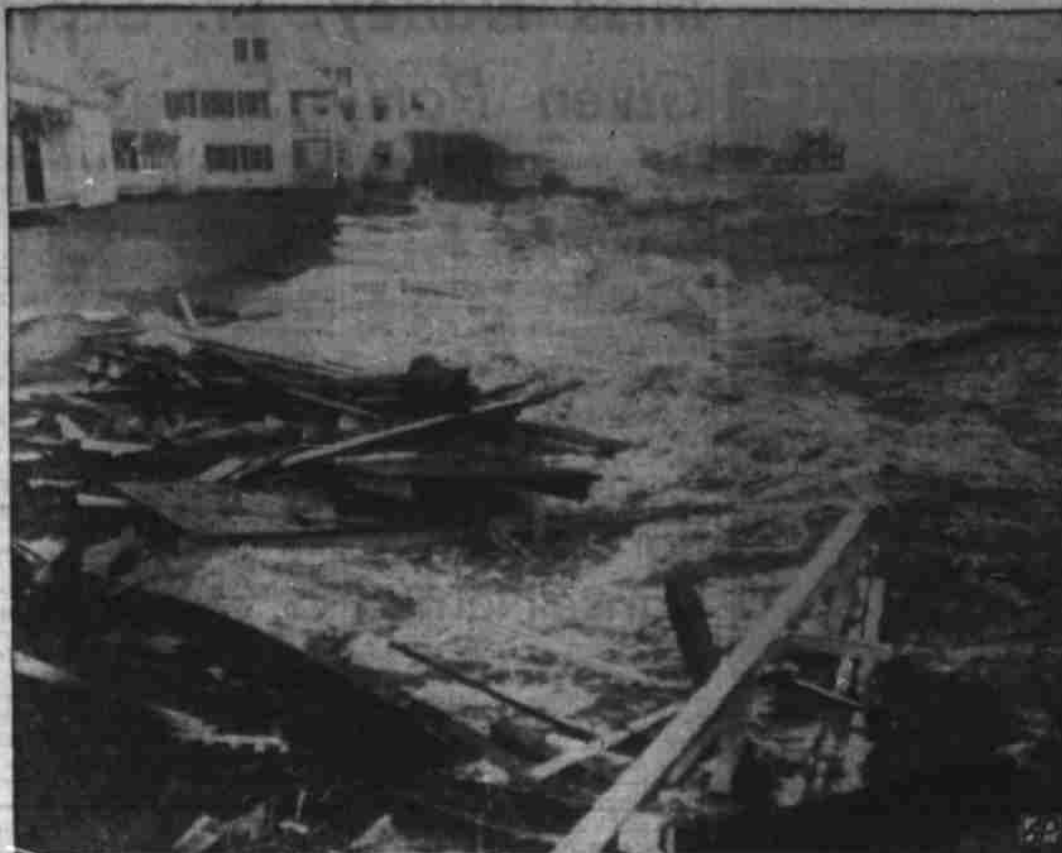
IONE HITS CAROLINA COAST WITH FURY Cottages along the Bogue Sound took a severe lashing
