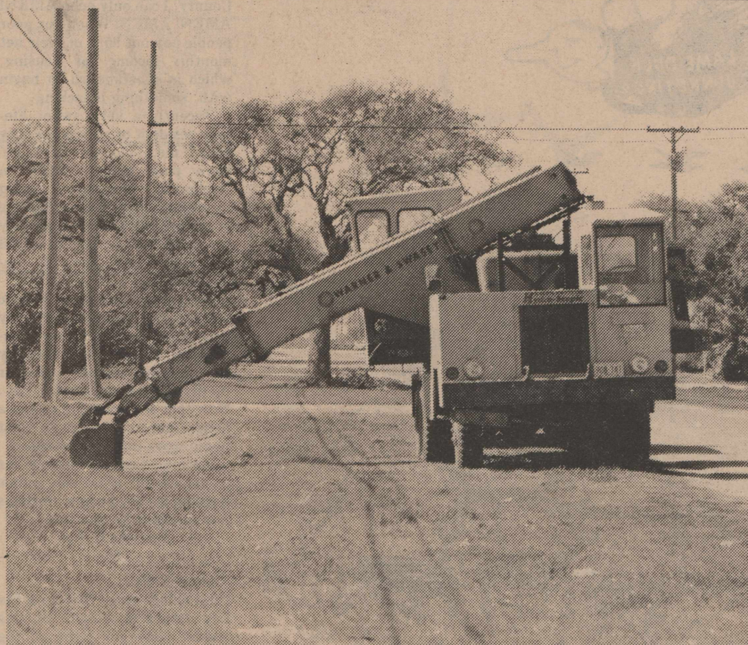
DIGGING IN. Spring is here at last, and the county road crews were on the job last week to begin the recovery from one of the wettest and all-around worst winters in memory. This ditch was getting a new bottom courtesy of this monster machine on a side street off Fulton Beach Road in Fulton. Hopefully, it won't be tested any time soon.
