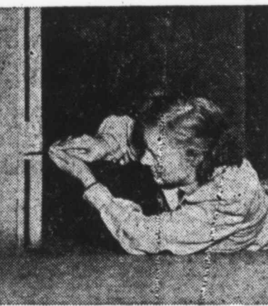
Wherever there are doors children will swing on them, hence the sag. Photo demonstrates the method of prying the screwdriver in taking the sag out of a door.
