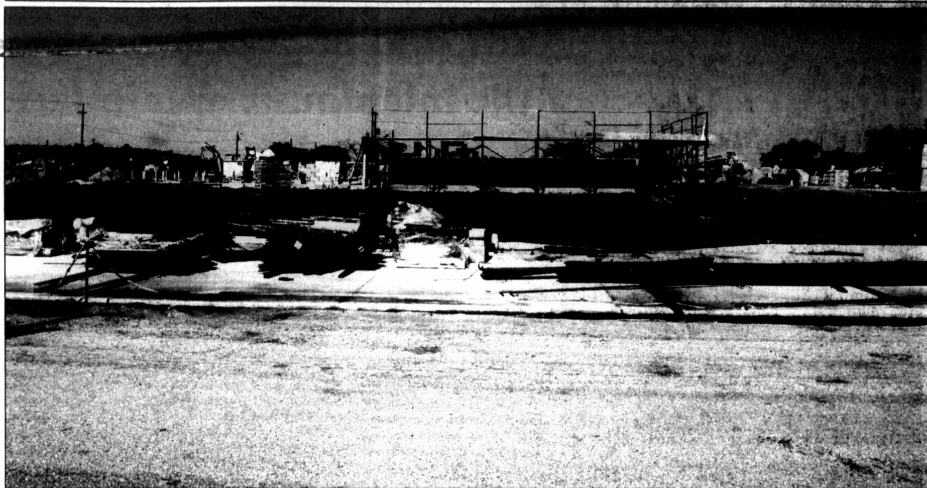
STARTING TO RISE — The construction of the new law enforcement center for Mitchell County took a different turn this week, up. The new site of the jail is across from the Mitchell County Sheriff's Office on Pine Street.
