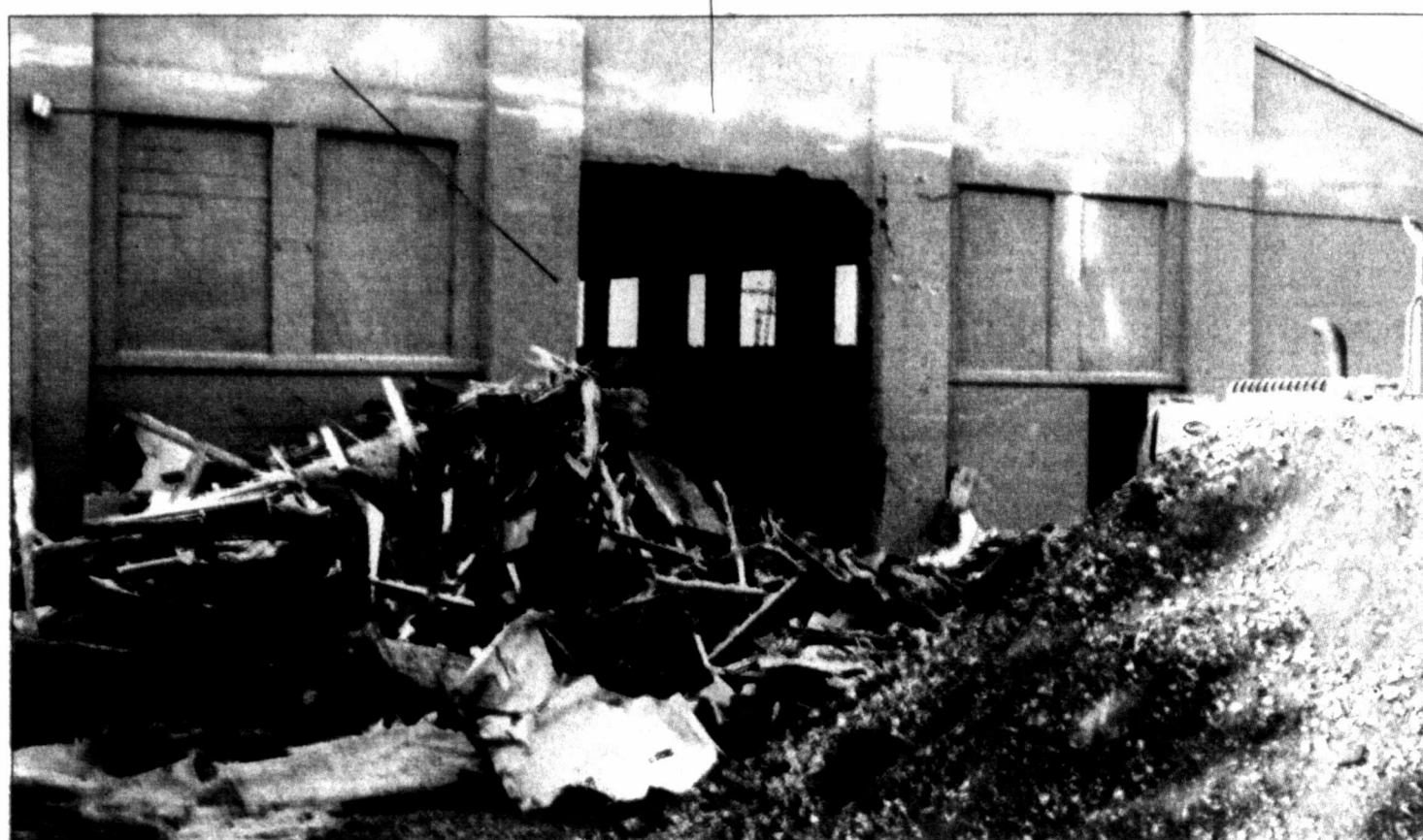
OUT WITH THE OLD... As the saying goes, the old must go to make room for the new. Construction on Loraine's new school has begun by way of demolition of the old gym, seen here. Crews have begun demolition on several of the buildings on the campus.
