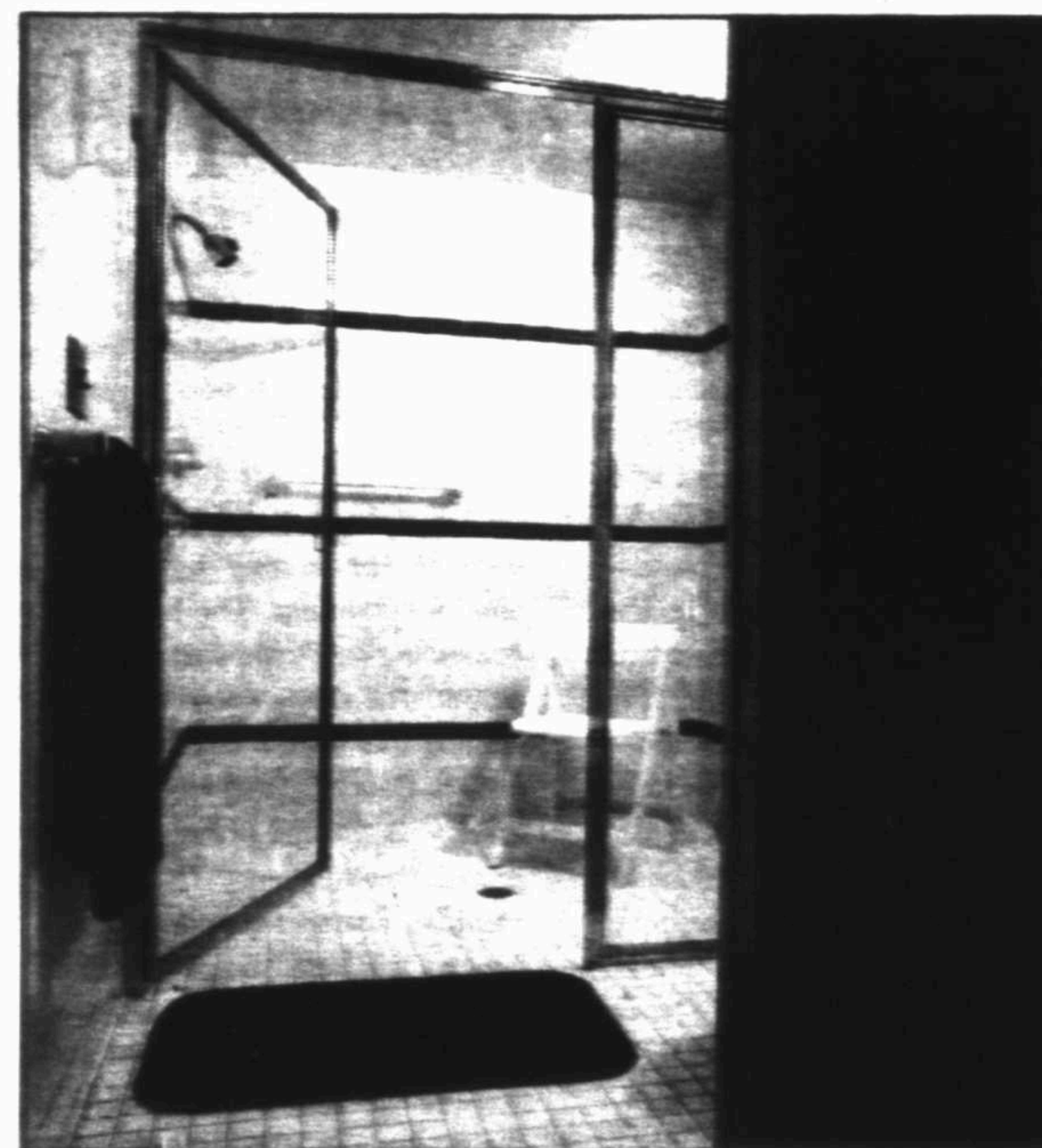
The all-tile wet room above allows a wheelchair to roll right into the shower through the extra-wide door. The floor slopes slightly to the drain.
