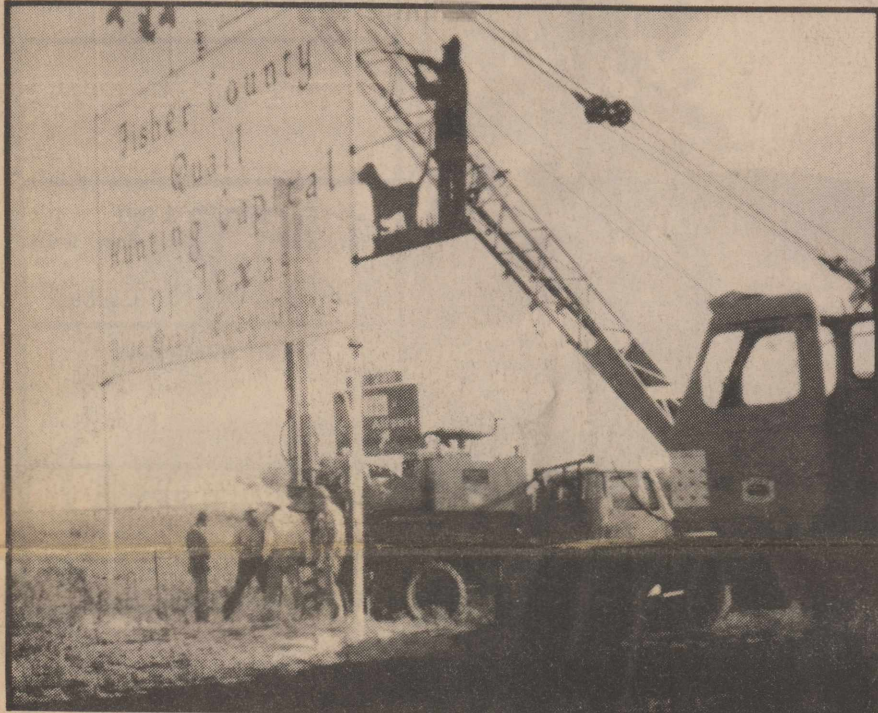
SIGN INSTALLED: A new sign hailing Fisher County as the 'Quail Hunting Capital of Texas' was recently installed on the Robert Nemir farm located near I-20 near Sweetwater. Sign was made by Joe Hull and installed by Midwest Electric Coop and Fisher County crews. The sign invites interested persons desiring additional information to write 'Quail, Roby, Texas'.
