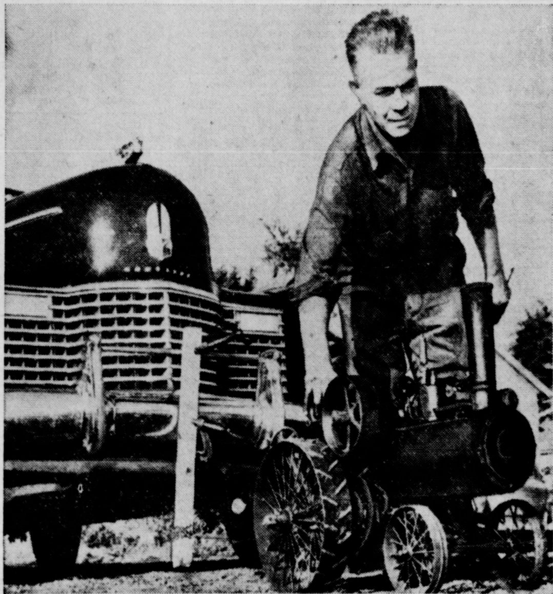
LITTLE BUT MIGHTY —Grant Goodfellow, a garage owner in Grand Rapids, Mich., is demonstrating an invention of his own. It's a working model steam engine which can pull a 4750-pound auto. The engine, weighing less than a hundred pounds, is complete in every detail from a hinged firebox door to the tiniest valve necessary to help make it run.
