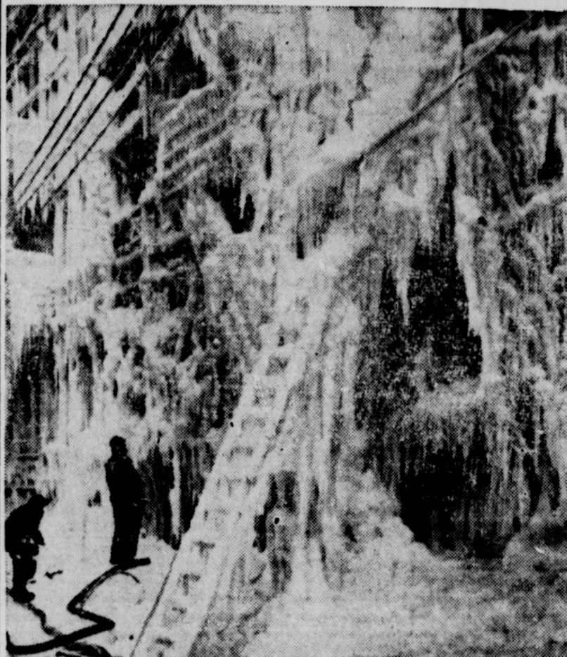
ICE HAMPER FIRE-FIGHTERS . . . In sub-zero cold which brought frostbite and exposure to scores of fire-fighters, fire in Akron, Ohio, downtown business area burned with a loss officially estimated at $500,000. The above photograph shows part of the ice-encrusted buildings in the fire-gutted block. It was Akron's biggest fire in 25 years in which the business section was endangered due to freezing temperatures.
