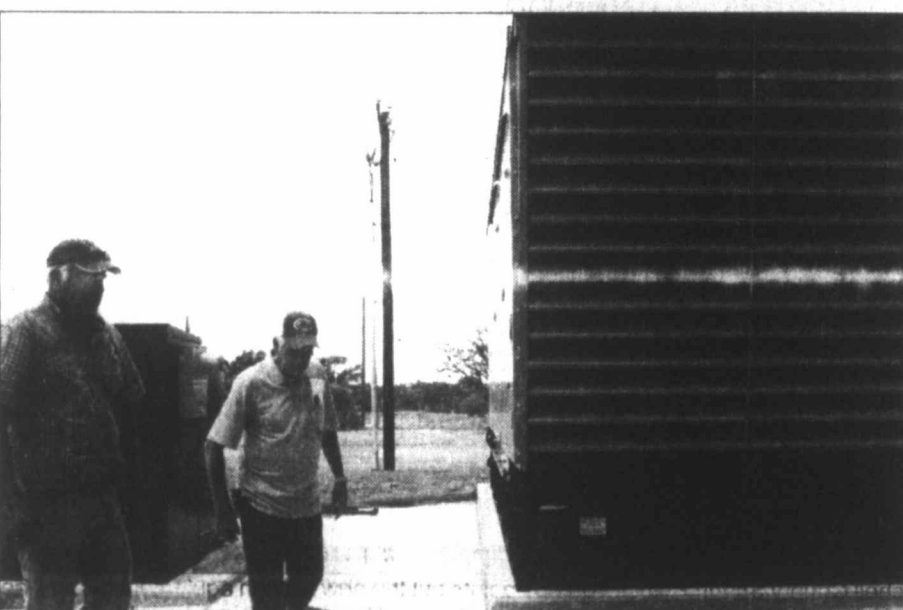
POWER UPI Ray Ritchey and V.O. Kuhn check out the big generator...
