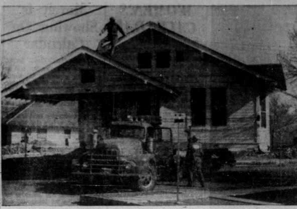
HOUSE BEGINS JOURNEY—This frame house began a journey from Snyder to Clairemont yesterday, as men and equipment of W. K. Bingham and Sons went into action. The house, located at 2112 Twenty-seventh Street, had been at that location for about a century. It had been owned by the E. E. Snyder family.
