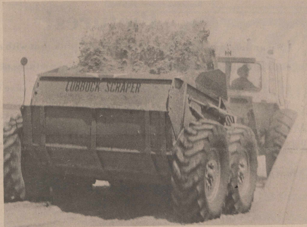
MOVING THE HILLS -- After knocking down the steepest part of the hills, tractors pulling Lubbock Scrapers, which augers the sand up into a loader, comes along and finishes leveling off the hills. Behind the scrapers, a land leveler comes and puts the final touches of leveling before the fertilizer is added.
