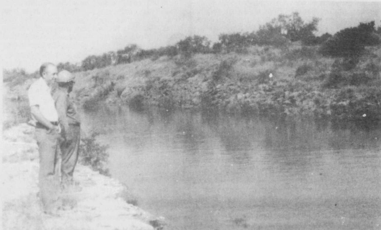
TESCO OFFICIALS, Bruce Moore (left) and Jim Luera (right) check the spillway at Lake Champion after recent heavy rains. The water was running out of the service spillway for the first time since the lake was built back in the mid 1950's.
