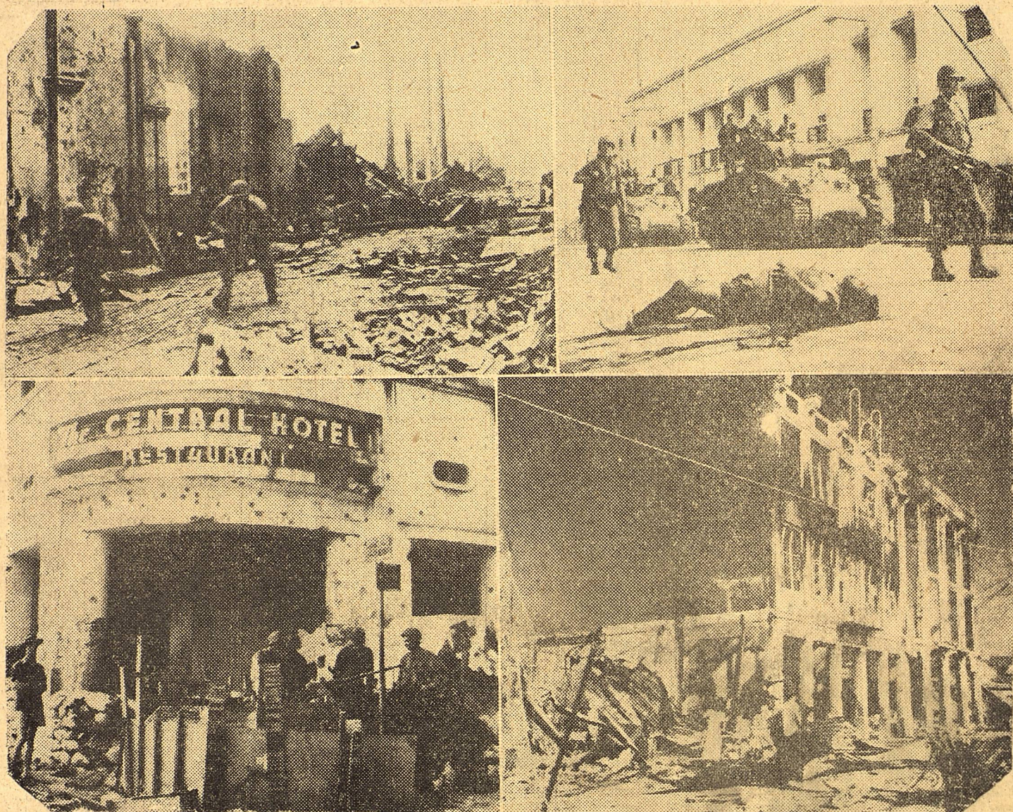
Through flame-blackened ruins of this Manila building, upper left, these American infantrymen crouch low as they pursue the retreating Japs. Bitter house-to-house fighting still rages in the city. Upper right pictures a Jap, sprawled grotesquely in death, in a Manila street as American medium tanks and infantrymen advance past shell-pocked Far Eastern University building. Lower left pictures invading Yank infantrymen inspecting a knocked out Jap machinegun nest set up at a street corner in front of Manila's Central Hotel. Lower right shows that only one wall is left standing of this Manila building, set ablaze by retreating Japs, and smoke from other fires still darkens the sky above the city. (Photos by Stanley Troutman, NEA Photographer for the War Picture Pool). (NEA Telephotos).
