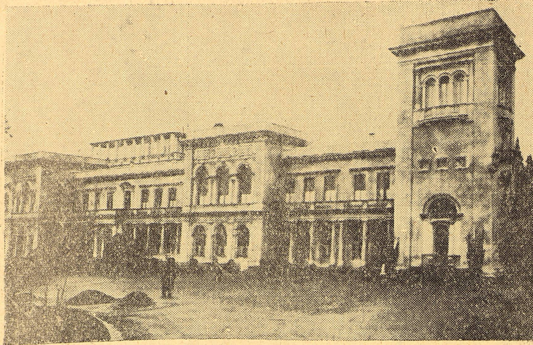
A general view of the palace at Yalta, Crimea, Russia, where the "Big Three" conference took place. President Roosevelt's quarters and conference room is on the ground floor in the right wing. (Signal Corps photo from NEA Telephoto).
