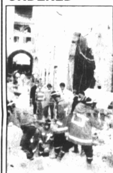
Firefighters work to remove debris after a car-bomb went off, killing five people at the Uffizi Museum in Florence's historic center in this 1993 file photo. Four reputed mobsters were ordered arrested Saturday on charges of masterminding the blast.
