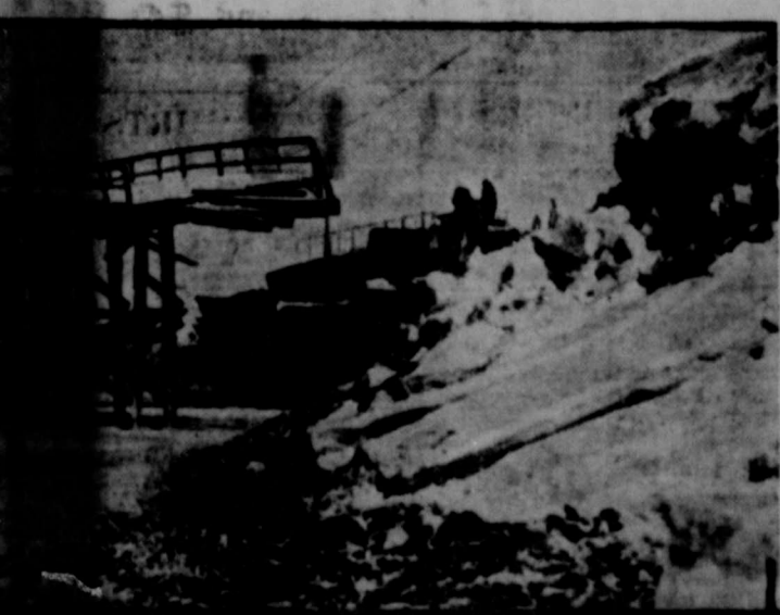
The railroad bridge at Hudson, Wis., over the St. Croix river which was damaged by a cave-in of the river bank thought to have been caused by skunks tunneling under the bank. In the background may be seen the wreckage of the Willrow River Power company's plant which was completely destroyed by the cave-in.
