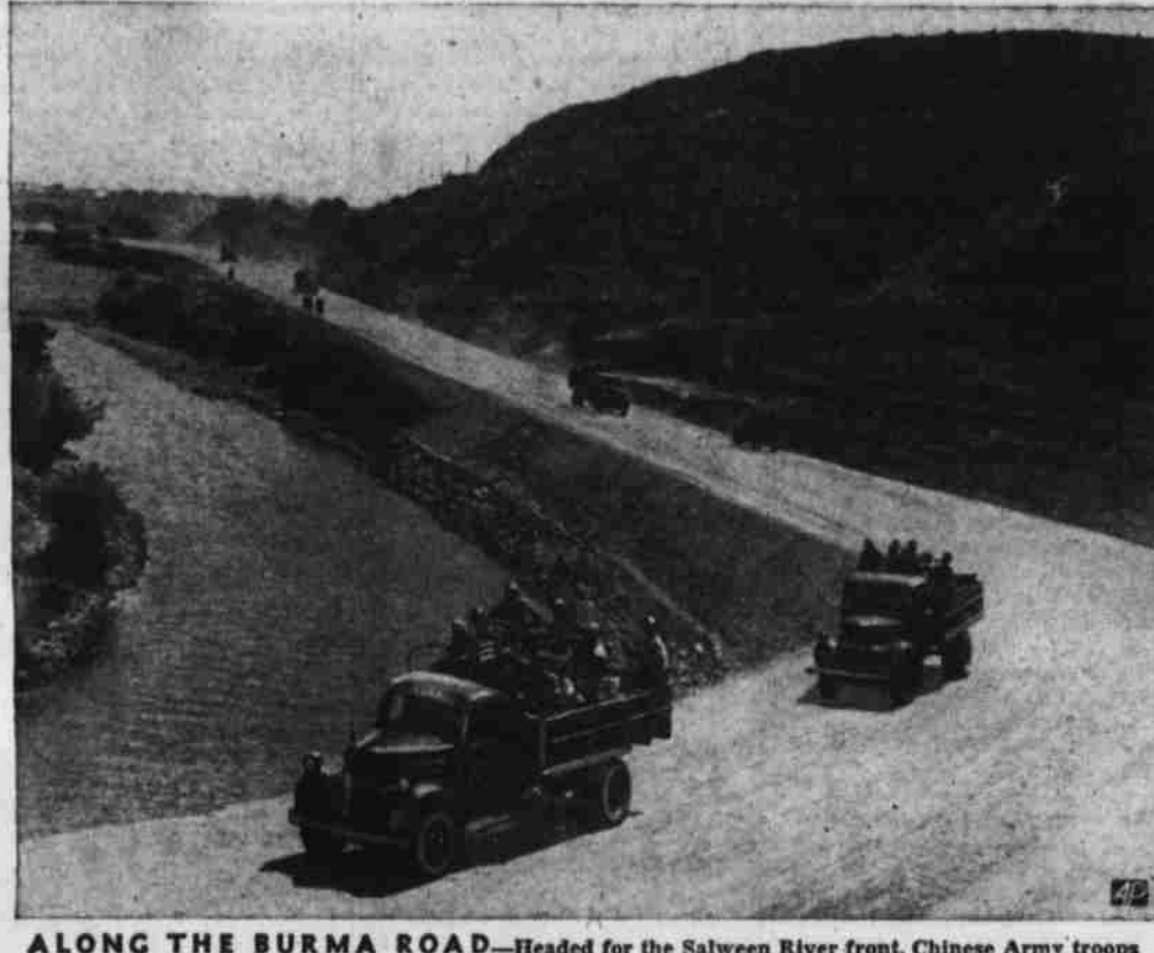
ALONG THE BURMA ROAD —Headed for the Salween River front, Chinese Army troops travel in motor convoy down part of the Burma road in company with American engineers.
