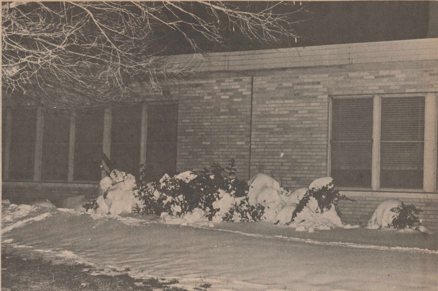
SNOWY SENTINELS -- keep guard over vacant H. P. Webb Elementary School building as vacationing students prepare to celebrate the passing of a decade. While winter's icy
