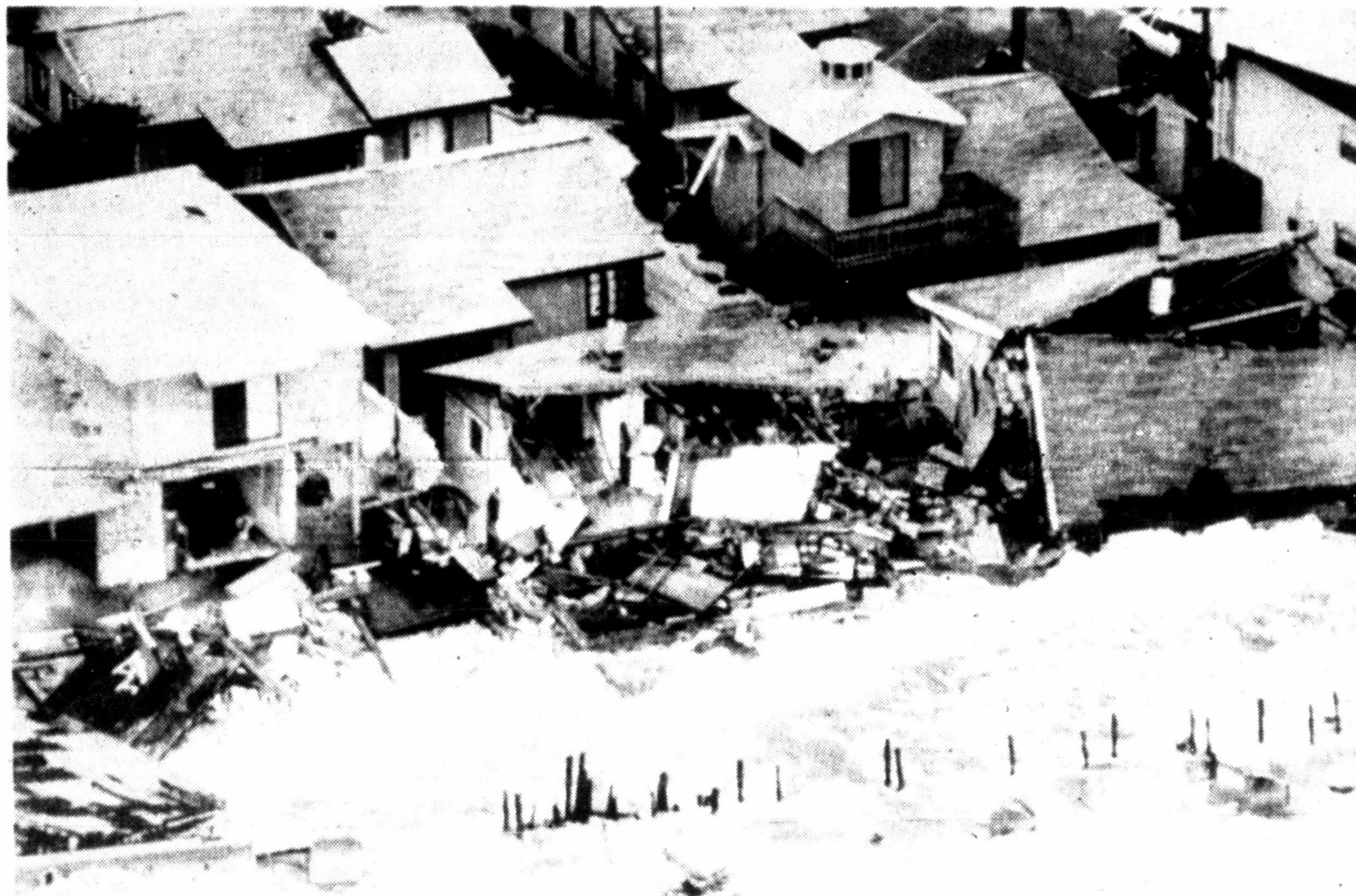
HOMES DAMAGED —Although Hurricane Elena didn't hit the coast of Florida, extensive damage was caused when storm tides sent surf crashing into beachside communities.
