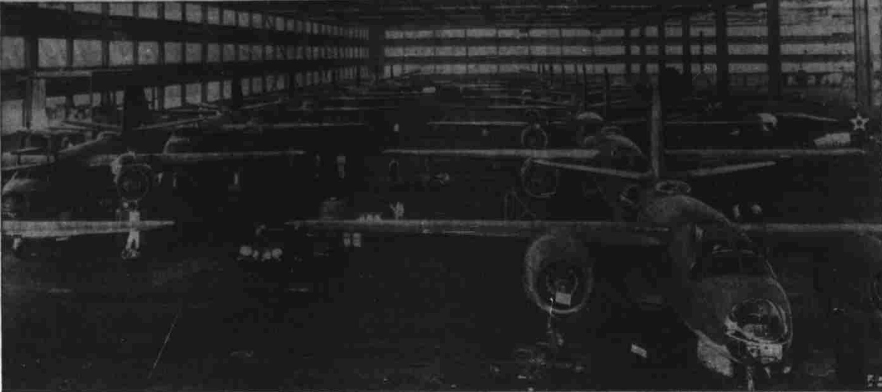
SIGHT FOR ALLIED EYES TO SEE —Powerful Army B-26 medium bombers are getting their final touches at a Baltimore plant of the Glenn L. Martin company, which is under mass production in a speed-up for defense. These speedy, heavily-gunned planes weigh 13 tons and pack self-sealing fuel tanks and power turrets.
