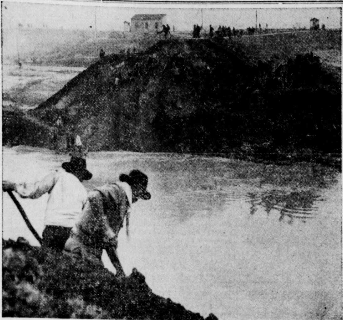
FILLING A BIG GAP —Farmers left their normal chores and worked around the clock to fill the gap opened in an embankment by flood waters of the Panaro River, near Camposanto, Italy. Days of steady rain caused damage running into millions of dollars.
