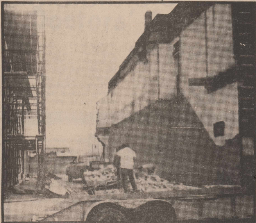
TEARING DOWN OLD DRUG BUILDING: The condemned building beside the WTU Office in Roby has been torn down to make way for a new park to be built there in the near future.
