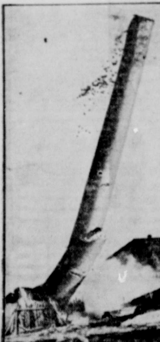
Cracking as it falls, a 35-year-old, 135-foot coal mine smokestack at Norway, Mich., is caught by the camera as it topples to earth just after a dynamite blast had ripped away its foundation.
