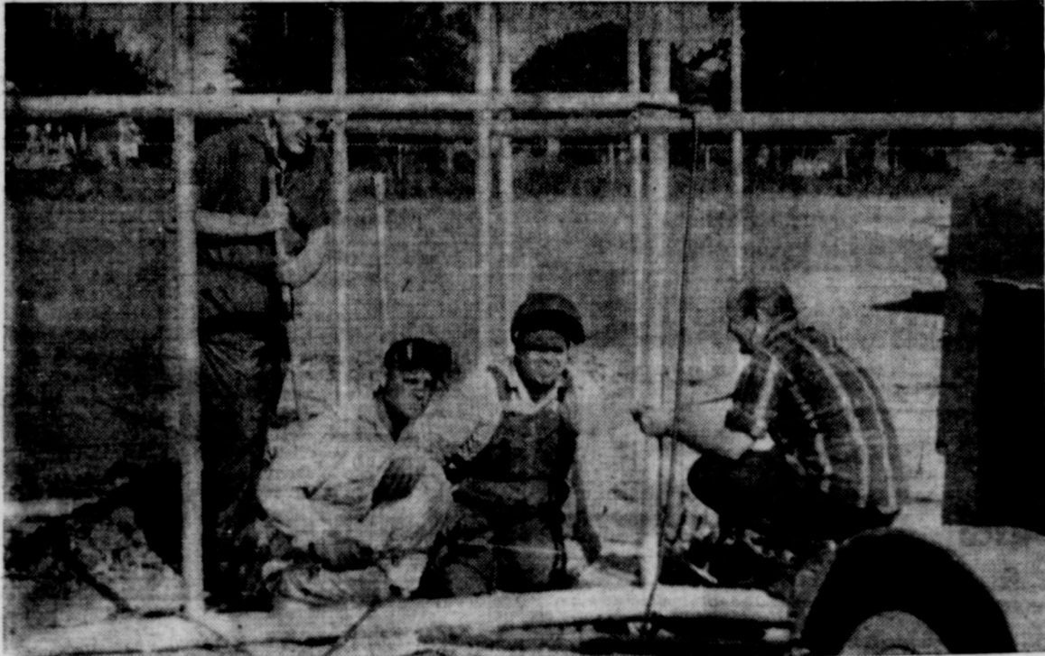
VOLUNTEER WELDING at the girls' softball practice court was plentiful this summer. Here John Morgan, Jerry Burden, C. J. Lippard and Jim Sullivan
