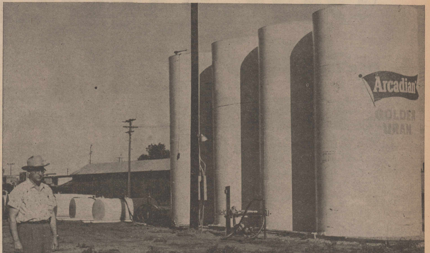
Pictured above are the new storage tanks for Arcadian Sol-U-Phos liquid fertilizer that were erected by Warrick Feed Store recently to handle this product.
