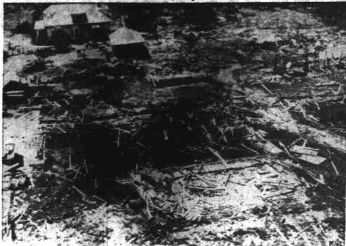
TORNADO WRECKAGE —A tornado struck this farmstead three and a half miles southeast of Fairfax, Mo., splintering all the buildings except the house and garage shown in the upper left of picture. More than a score of persons were injured in this extreme northwest corner of Missouri, and in Nebraska, Iowa and Kansas where the twisters hit. (AP Wirephoto)
