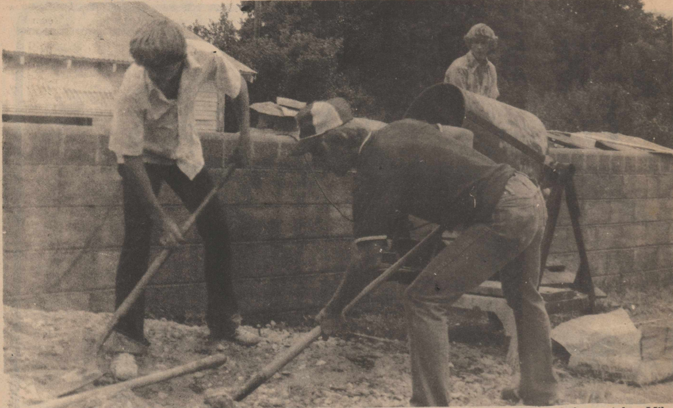
ROBY FFA PROJECT: The Roby FFA Ag-Mechanics class participated in a cement project where they poured a driveway and walk for J.T. Pope. Left to right, Mike Wilburn, Mike Terry and James Putnam.
