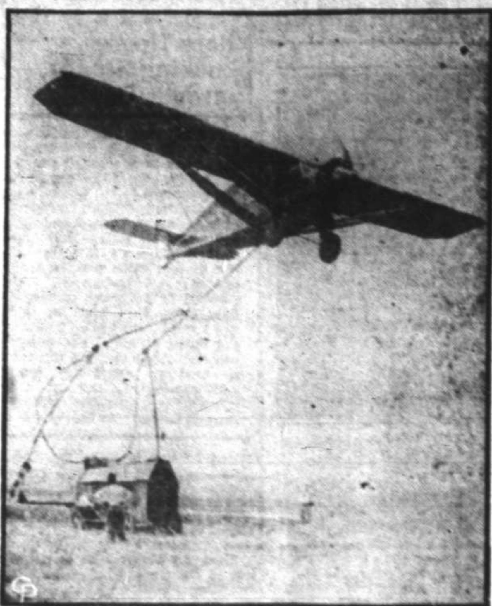
Speeding up of the air mails is expected to result from the perfecting of the Cabot aerial pickup device (shown above) being demonstrated for the first time. The novel invention permits a plane in full flight to pick up a mailbag from the ground. Roger Wolfe Kahn, son of the banker, piloted the plane in its test at M'Chel Field, N. Y.
