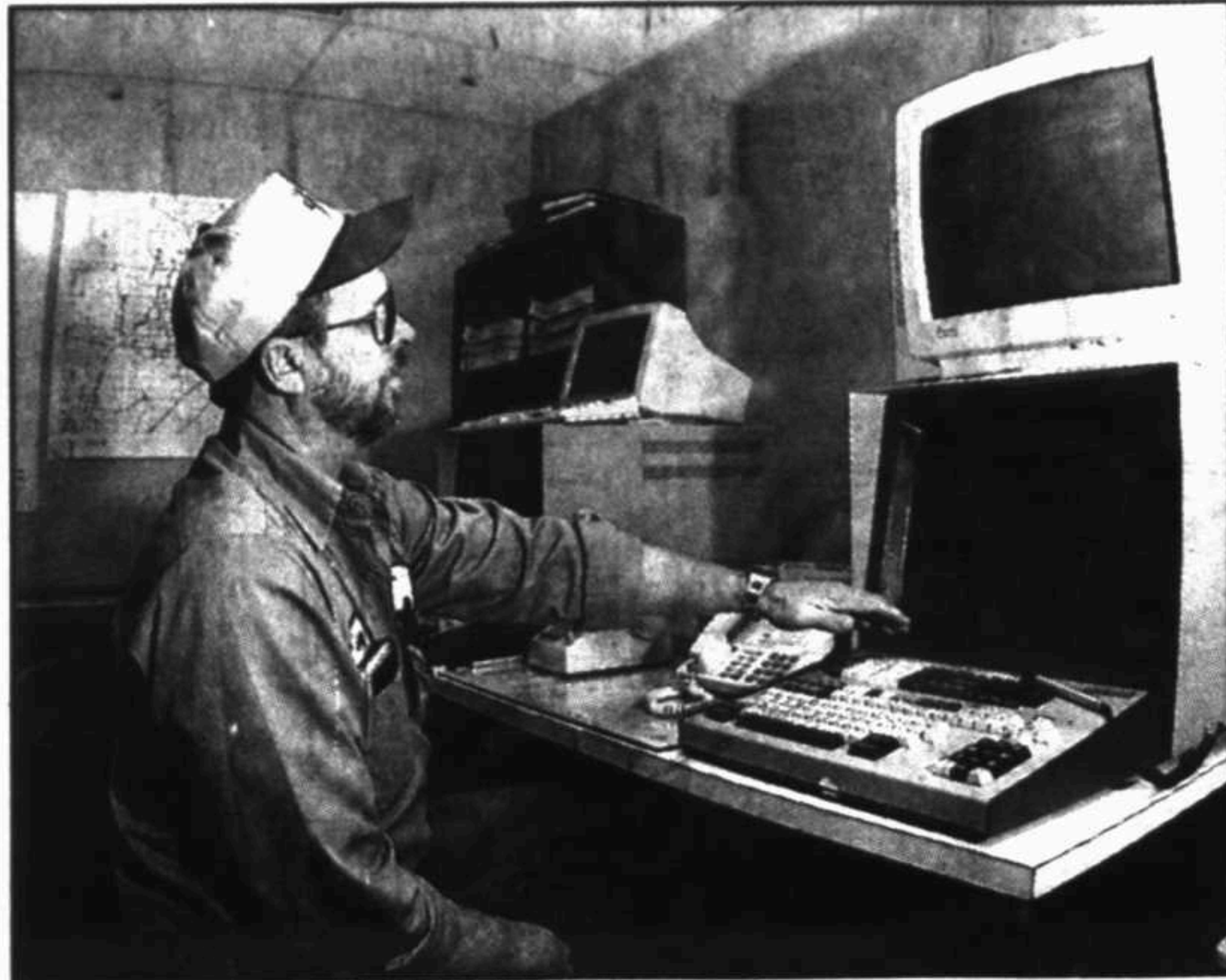
Gary Reid, a technician with Caprock Electric, oversees the field data monitoring system of the utility. The system, which monitors 19 substations, will be upgraded to become Y2K compliant, Reid says.
