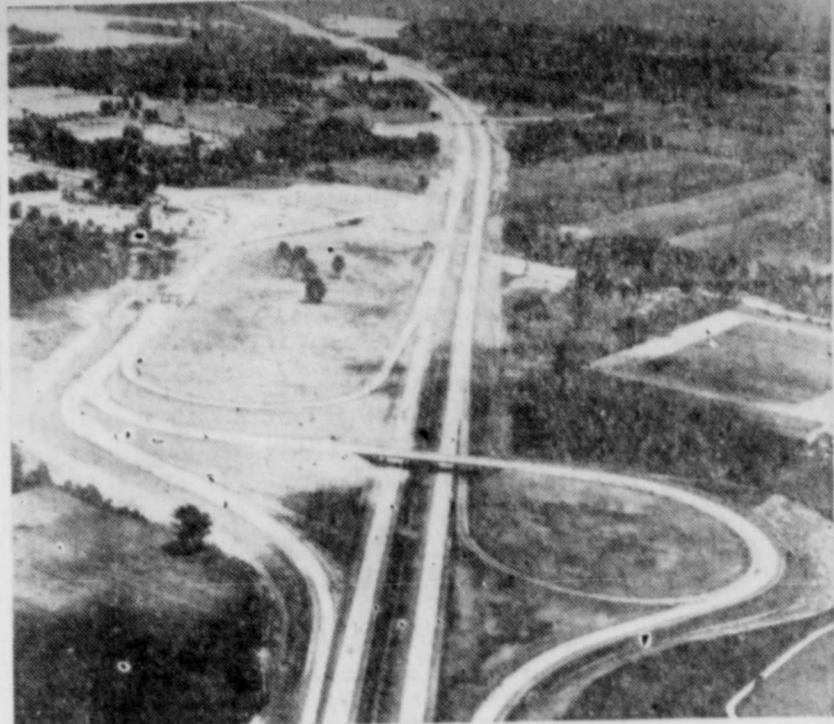
Aerial view of Niles-Youngstown interchange, seven miles west of Youngstown. Route 18 crosses underneath. Toll plaza is at left center. Upper left, Meander Creek reservoir. In all, there are 15 interchanges and two state line terminals.
