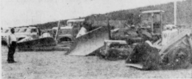
Maintenance. Big dump trucks and snow plows have two-way radio. There is a maintenance shop with 15 full-time employees every 30 miles. Turnpike has more than 100 pieces of self-propelled maintenance equipment.
