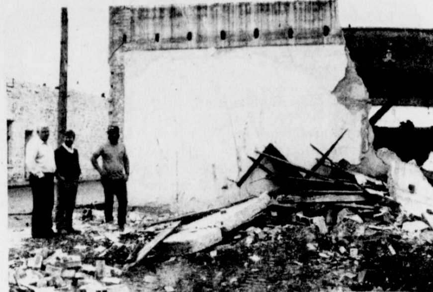
And they all came tumbling down: The Winters Enterprise office got a nice surprise last Monday. The old buildings that occupy the lots behind Main Drug and The Winters Enterprise office have been cleared. Thanks to Guy Contractors, Main Drug and the Chamber of Commerce, Winters is a lot more attractive. Let's all help make Winters nicer and more attractive for the birthday. Pictured left to right are, Gary Moore, WTU; James Cross, Main Drug; and Barron Guy, Guy Dirt Contractors.
