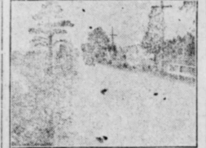
Road Treated With One Application of an Oil Emulsion—Automobile Traveling at Rate of 40 Miles an Hour, With No Dust Resulting.
