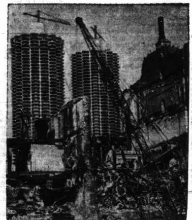
UP AND DOWN —Cranes are instruments of construction and destruction in a Chicago area where Marina City is being built while other structures are razed.
