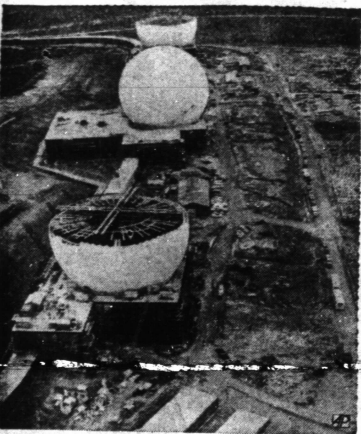
RISE TO WARN —Radomes near completion at a ballistic missile early warning station at Flyndales, England. They'll operate in conjunction with U. S. system.
