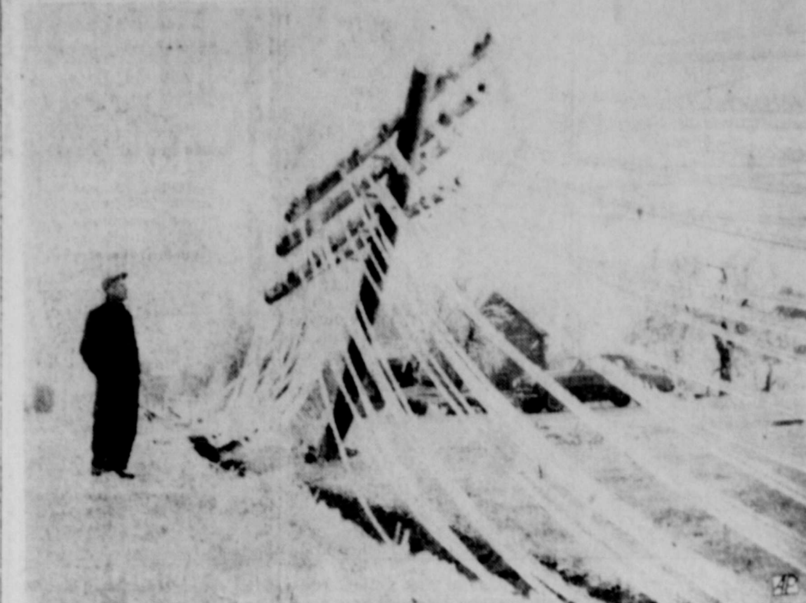
ICE DOWNS TELEPHONE LINES —F. W. Gray of Howe, Tex., surveys damage to telephone lines in the city just south of Sherman, Tex., after they were pulled down by a coating of ice Feb. 1. Fifty-four or more towns in the North Texas area are isolated from telephone connections. Southwest Bell Telephone Company said a total of 747 circuits are out and some 455 poles are down. Power failures left three towns without water.
