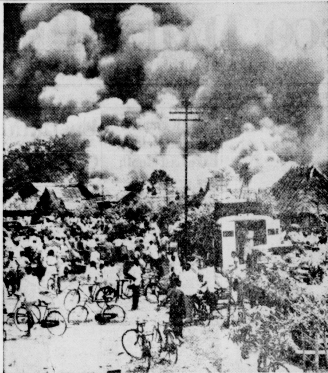
THE MONSTER OF FIRE —Crowds in Singapore watch in terror and despair as hut after hut in the Kalland district goes up in flame. Whipped by stiff breezes, fires like this are a constant threat in the shantytown where refugees from Red China come to live under Western protection
