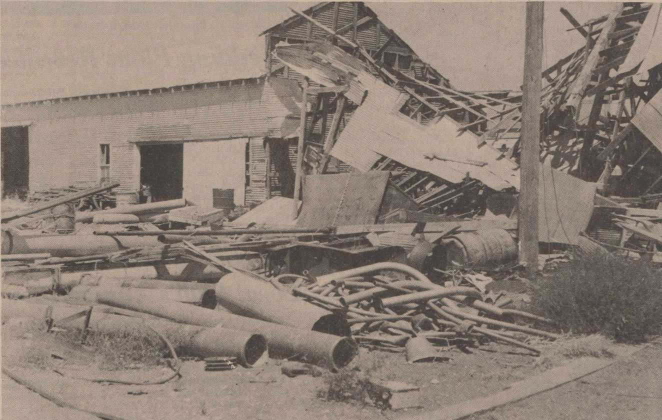
A terrible Eye Sore is the old gin right on the Hiway 70 - People driving through Olton must be shocked at the apathy.
