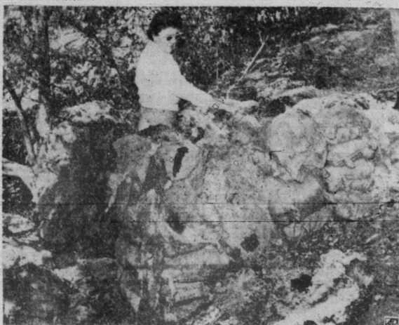
NOBEL WINNER'S FALLOUT SHELTER AFTER FIRE—Mrs. Betty Strobel looks over the $30 fallout shelter built by Nobel Prize winner Dr. Willard F. Libby which partially survived the raging brush fire that destroyed his and other homes in the Bel-Air district of Los Angeles. Railroad ties covering the sandbags in the backyard shelter were burned off, but the walls were only slightly affected. Libby says he still has faith in the shelter design as a protection against fallout. (AP Wirephoto)
