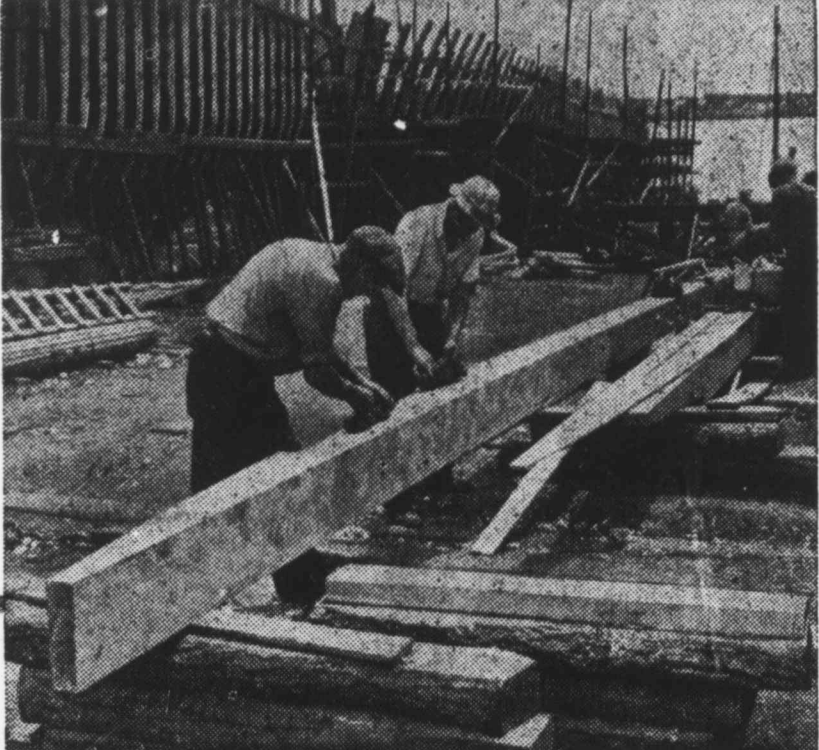
Two shipwrights work on a keel here. In the background are two hulls in various stages of construction.
