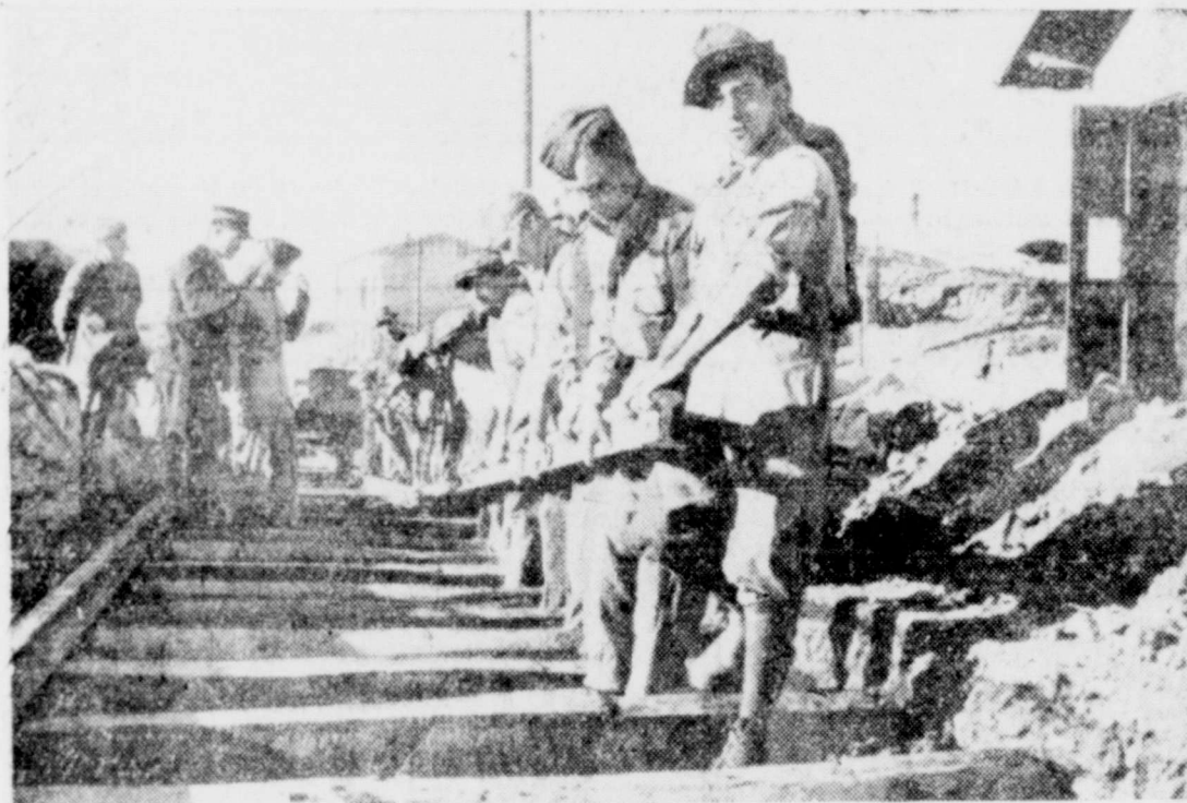
AFTER THE NAZIS—Working side by side with Eighth Army Tommies, men of Termoli, Italy, reconstruct stretch of railway. Here, they place 39-foot rail in position on ties.
