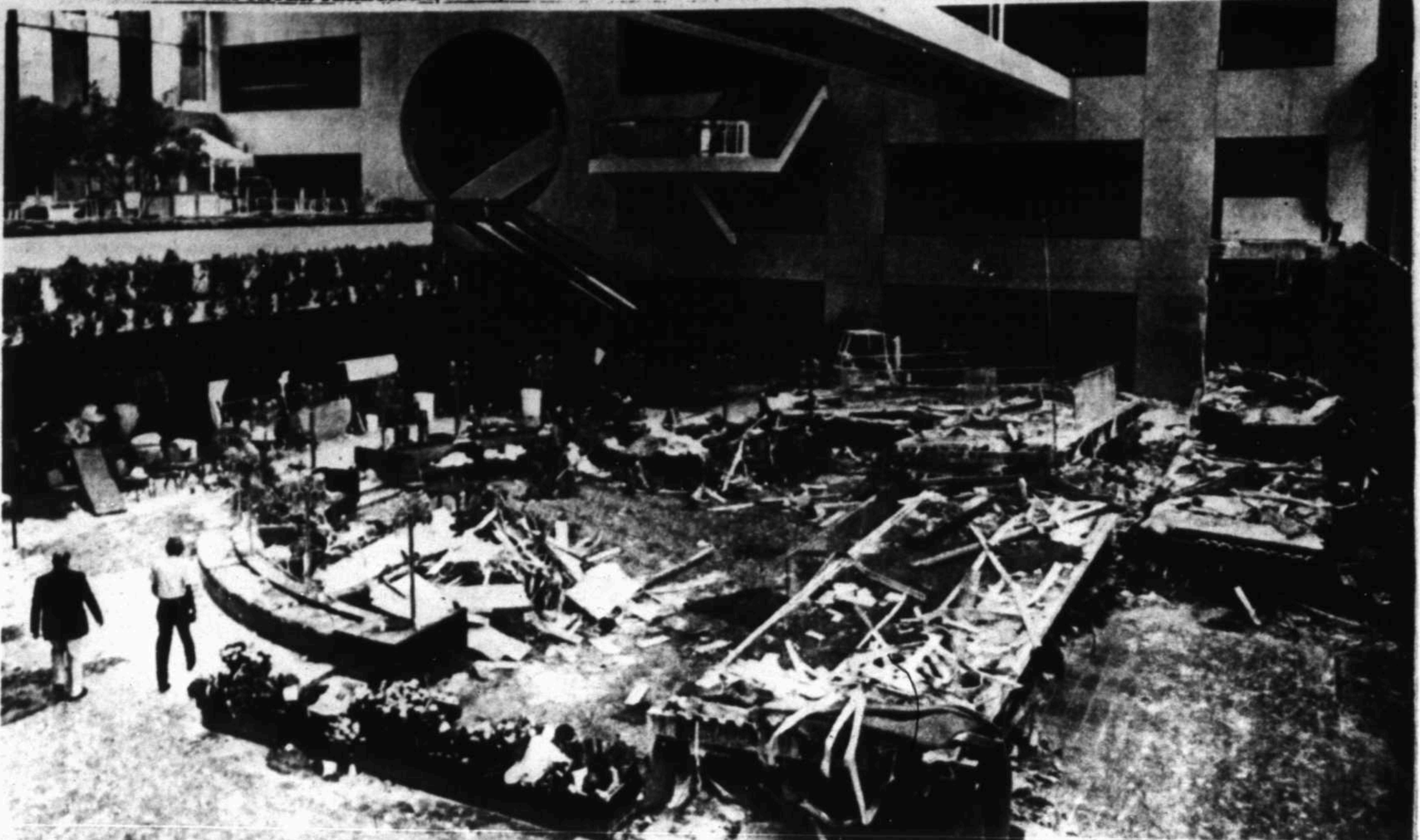
Two unidentified men walk through the lobby of Kansas City's Hyatt Regency Hotel Sunday scattered with the damage of Friday
