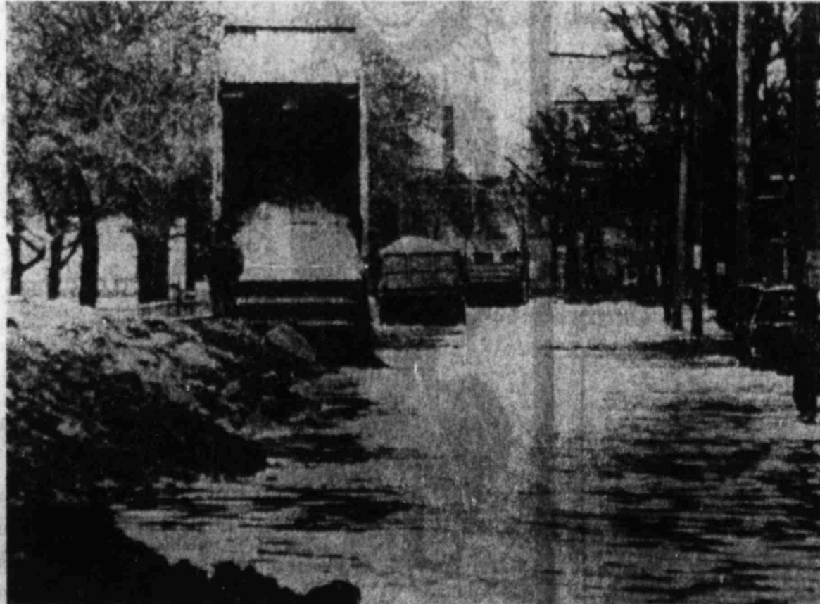
FLOOD WATERS PLAGUE PORT WAYNE—City workers build 7-foot-wide earthen dike Thursday to hold back flood waters from Spy Run Creek in Port Wayne, Ind. Spring flooding,
