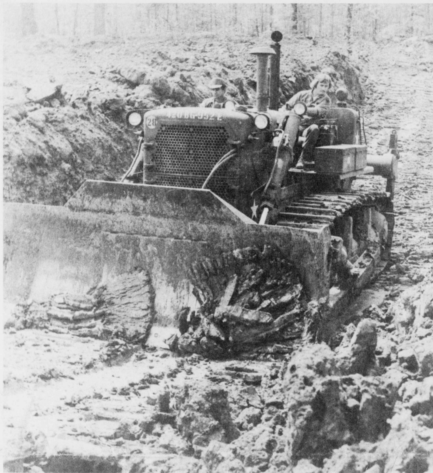
DIGGING OUT —The 952 Engineering Co. of the Army Reserve, Paris, covered the Bogata City Dump, then dug this giant trench for future dumping. The project was completed in one weekend, and the cost to the City of Bogata was limited to the fuel used by the equipment. (Staff Photo).
