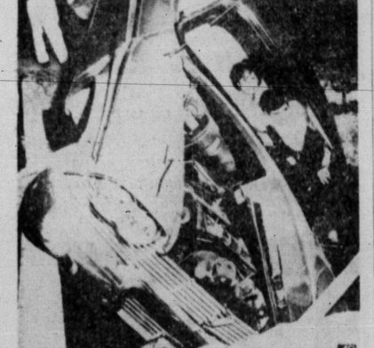
HELP—Mike Ocean, 20, right, and Francine Strauss, 18, wait for rescuers after their car had dropped part way into a sewer ditch excavation in Los Angeles. With the help of firemen and police, they were able to open the door and scramble to safety. Neither of the youngsters were injured. (AP Wirephoto)
