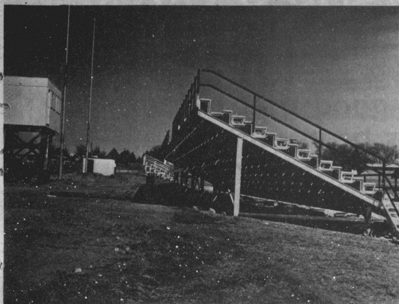
ALL-WEATHER TRACK CONSTRUCTION UNDERWAY --Workmen have already moved the visitor's pressbox and light standards at Benny Douglass Stadium west of Muleshoe High School, and are preparing to move the visitor's stands back several feet. The moves are being made to prepare for construction of a new all-weather track around the outer perimeter of the football field.
