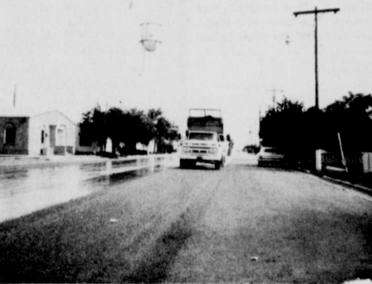
Paving contractors are shown sealcoating a portion of Avenue E. The City of Abernathy has contracted to have 22,757 square yards of pavement sealcoated in various parts of town.
