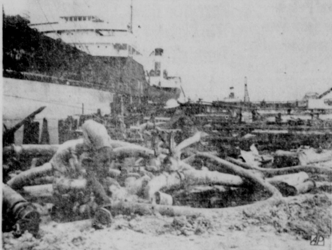
TEXAS CITY ONE YEAR LATER—Oil pipe lines for loading tankers were back in service within a month after the Texas City, Tex., disaster, April 16, 1948. Over a million tons of liquid cargo and sea-train dry cargo was shipped from the port in February, 1948, and amount only slightly below the overall tonnage figure for March, 1947, the last full month of operation before the disaster.
