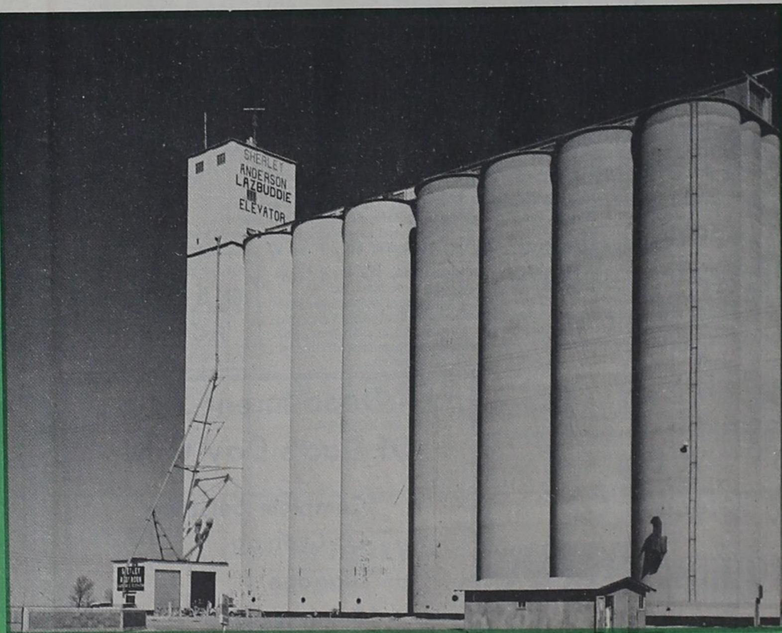
Sherley - Anderson LAZBUDDIE ELEVATOR
