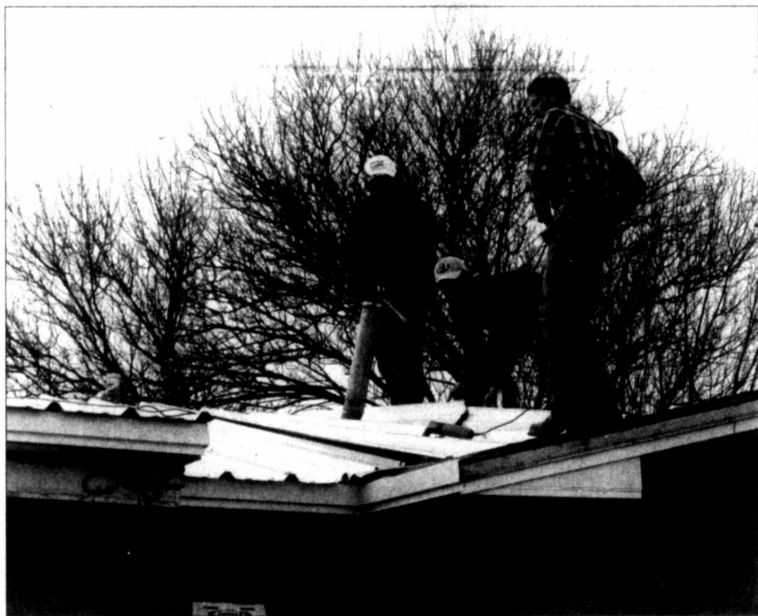
UP ON THE ROOFTOP - Workers from Ventura Construction secure new metal roofing to a home with funds granted to the Colorado City Housing Authority through President Obama's stimulus recovery program.
